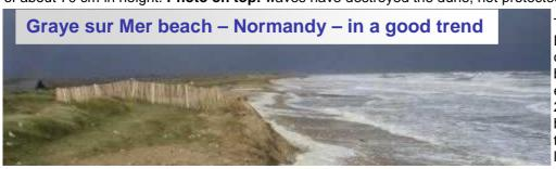
The eastern littoral part of the breach of La Valette, in Graye sur Mer town, is part of a coastline for which the average backward movement of the coast is estimated to 16,98 m for the years 1995-2004. From now, on this area is protected by 5 STABIPLAGE® works perpendicular to the coastline; they catch and stabilise longshore sediments: the last 2 works have
