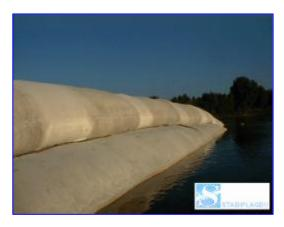
The **patented double-layered structure**: a permeable filter, covered with a resistant shell, makes it possible to ensure longevity in time of the shape of the work and its resistance to the agents of erosion: abrasion by sand, UV, hydrocarbons, various waste carried out by the currents or the tides.
